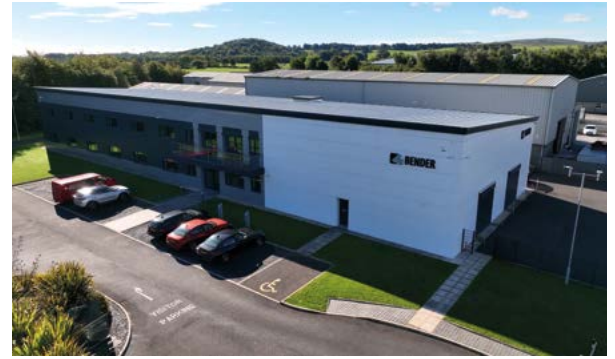
Bender UK's head office in Ulverston, Cumbria.
